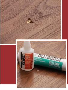
Applying Fill n' Finish Thin into a chipped-out area seals up the fibers of the ding preparing for the next step.
